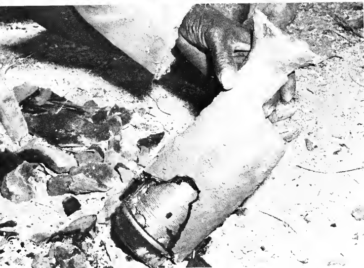
Casting brass in a clay mold — the "cire perdue" method
